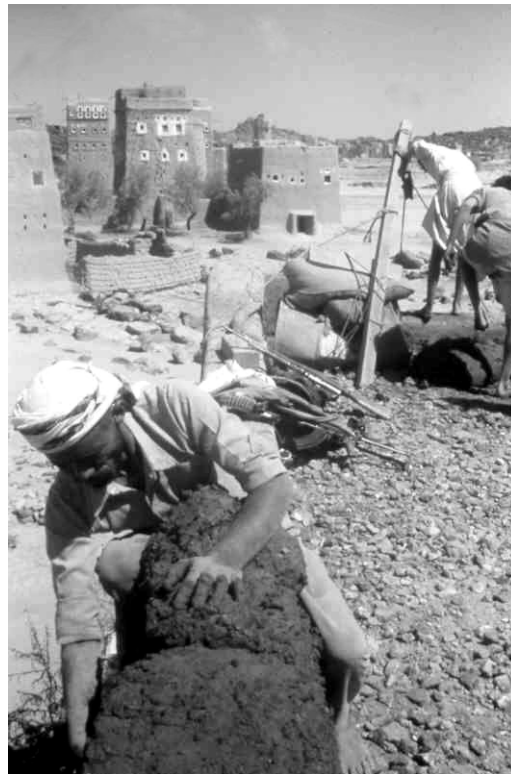
Right: Buildings were constructed of packed mud. Men mix mud and straw with their feet and the master builder forms it into walls. Left: A fortified house near Medina.
